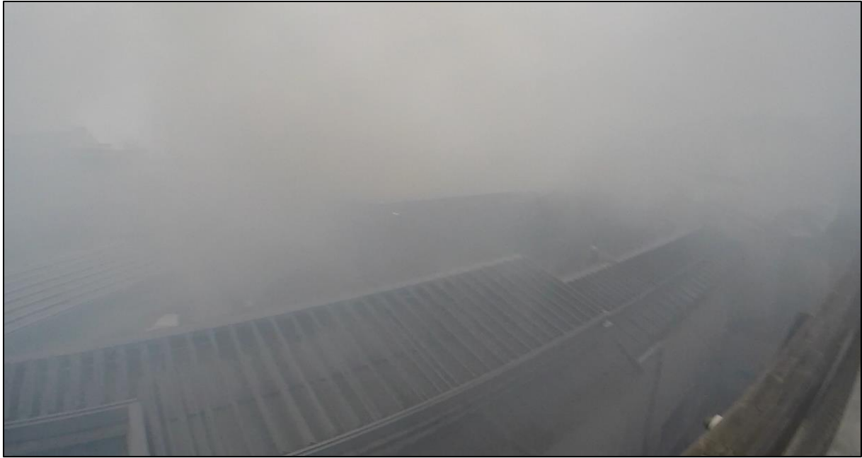
Image 4 View at the roof after putting down the flames of the built-up structure. (Picture: Davy Platteau)
