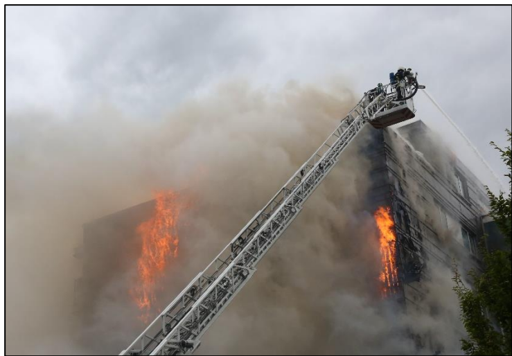
Figure 2 The cladding fire in Ypres. In some locations, the façade is “open” and flames are showing. In other locations, the façade is still “closed” and plenty of smoke is being produced. (Picture: Warre Saint-Germain)
