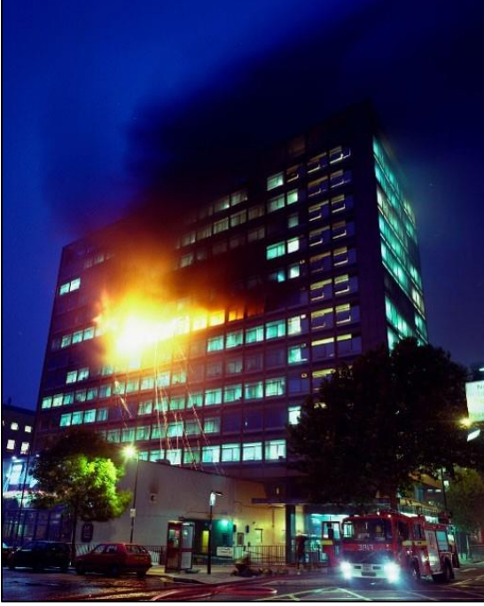
Şekil 2 Most of the windows have collapsed and flames exiting the building are a threat to the floor above. (Photo: London evening news)
