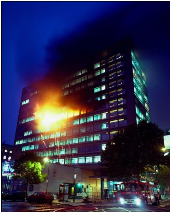
figure 2 Most of the windows have collapsed and flames exiting the building are a threat to the floor above. (Photo: London evening news)
