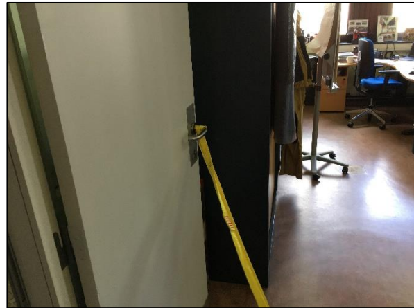
Figure 15 and 16 A lark's head knot is attached to the door handle or door knob. The door can then be closed with a quick pull and the firefighter keeps control of the door.
