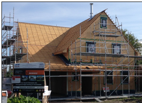
Figure 6 Construction of a wooden house. (Photo: Nathalie Van Moorter)
