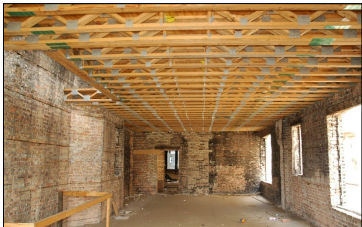
Figure 1 Wooden trusses (Photo: NIST)
