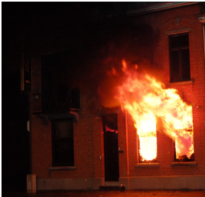
Figure 6 Fully developed fire venting from the ground floor windows of a house. (Photo: Nico Speleers)
