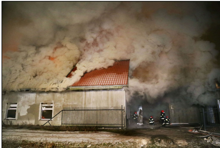
Figure 7 During this under ventilated fire, temperature inside is running very high. The overpressure inside will push smoke out. (© Photo: Zbigniew Wozniak)
