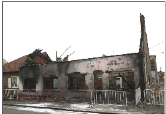
Figure 3 After a fire only the walls are left standing. Using crowd barriers and barricade tape the collapse zone is outlined. (Photo: Herman De Wit)
