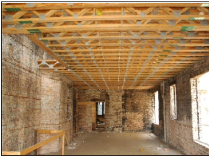
Figure 2 Wooden trusses (Photo: NIST)
