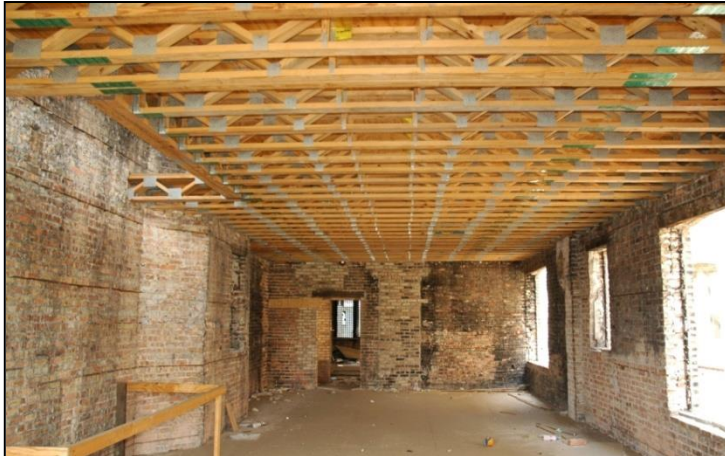
Figure 2 Travatura in legno (Photo: NIST)
