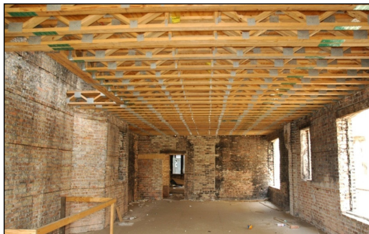
Figure 2 Entramado de madera (Photo: NIST)
