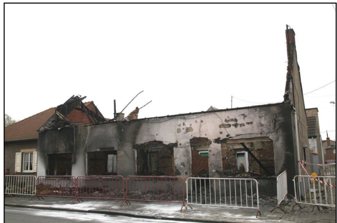
Figure 3 After a fire only the walls are left standing. Using crowd barriers and barricade tape the collapse zone is outlined. (Photo: Herman De Wit)
