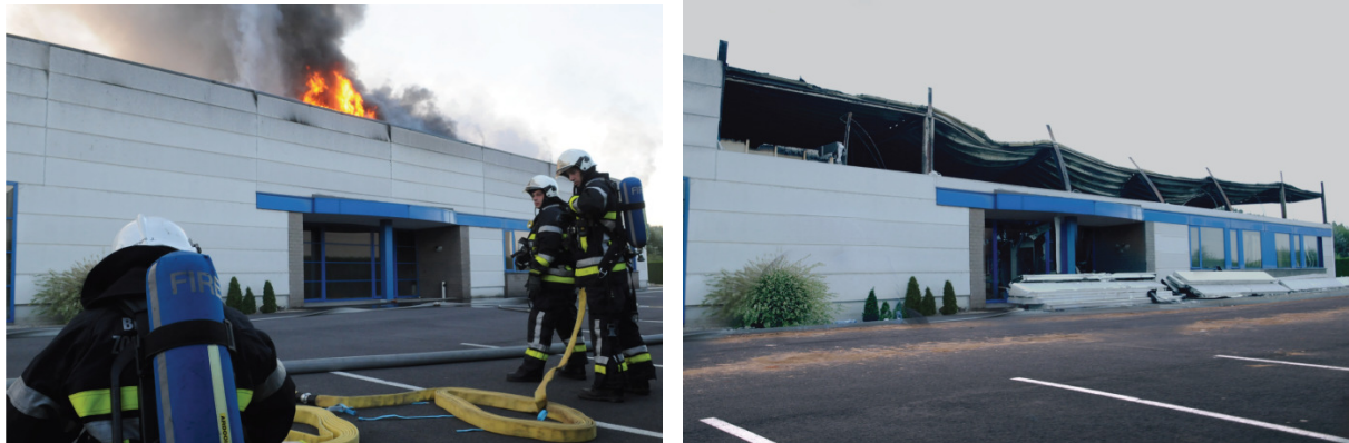
Figure 4 A fire in an industrial building made up out of prefab wall panels. Because of the risk for collapse, distance to the wall is kept. Afterwards, any loose panels are removed to eliminate the any risk for collapse. (Photo's: Peter Vangierdegom)
