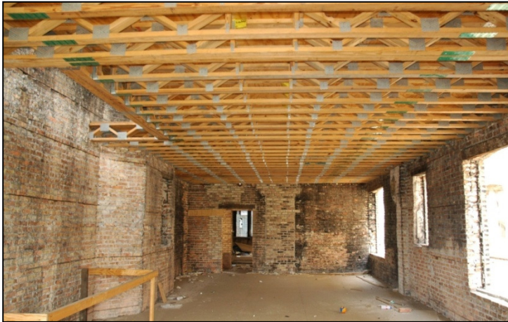
Figure 2 Wooden trusses (Photo: NIST)
