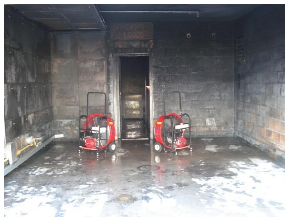
Fig. 9.11 Configurazione a forma di V in V-shaped configuration in a room where the side walls are too close to one another and the blowers cannot draw in sufficient air (Photo: Karel Lambert)
