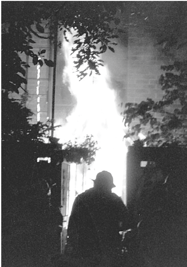
Fig 2.3 Exiting flames from the sliding window into the back yard. (Photo: District of Columbia Fire & EMS)
