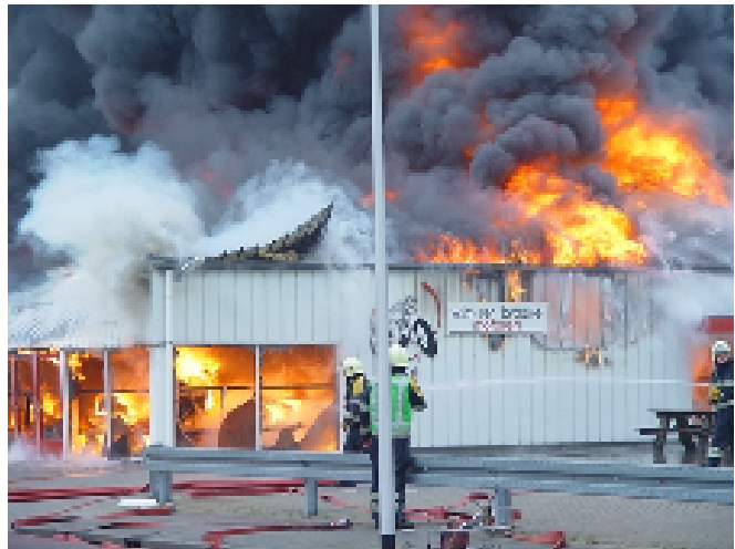
Fig 4.2 Exterior attack at a fully developed fire. Stability of the building is compromised and the building itself is beyond saving.
