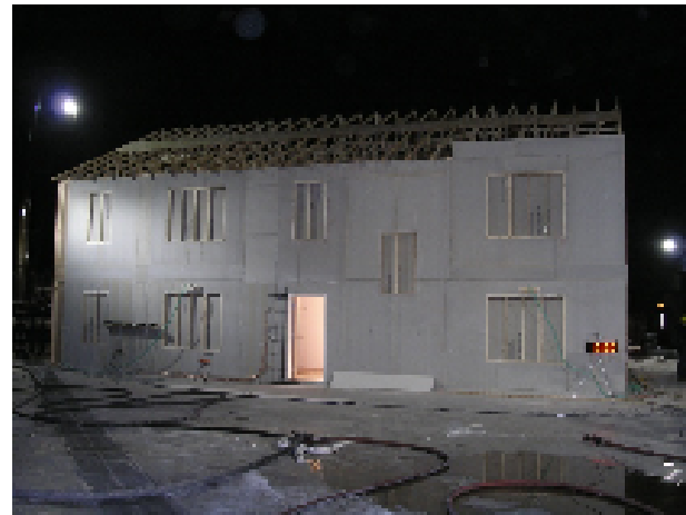
Fig 2.2 Two story house (297 m 2 ) (Photo: UL)
