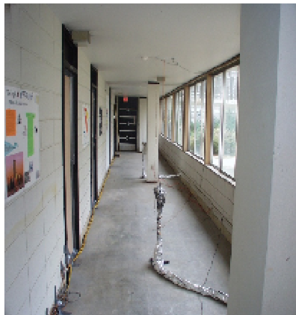
Fig 4.1 View on the hallway (Picture: NIST)
