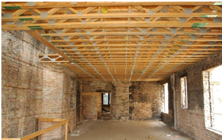
Fig 1.1 Travatura in legno. (Photo: NIST).
