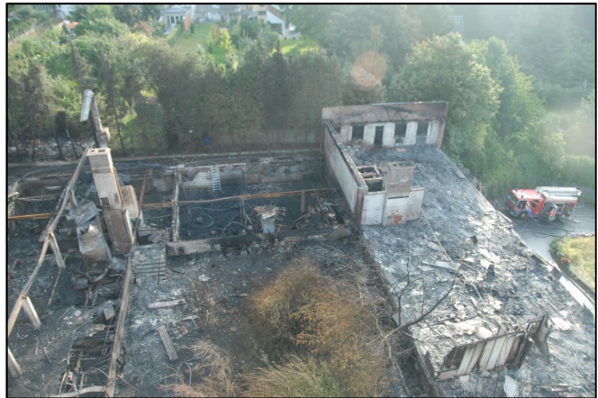
Figure 28 View on building C with building B to the right and what is left of the bush between buildings A and B. Notice the engine on the right side of the picture. Due to the slope of the terrain, the road is two floors lower than in front of the building at that point. (Picture: Robert Decock)
