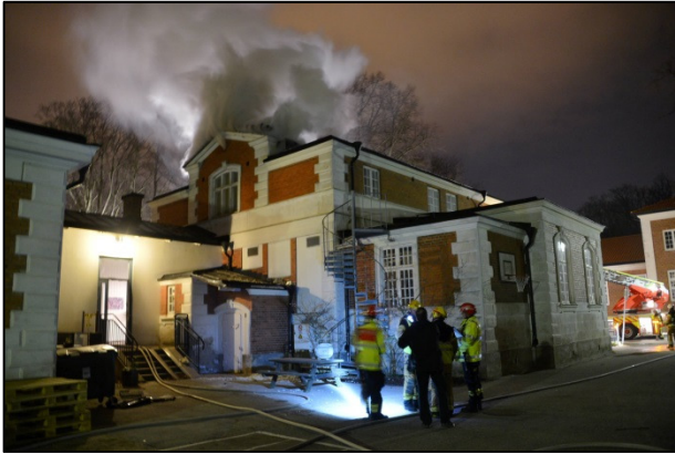
Figure 20 Fire in a school in Lund in 2009. The roof space is burning but due to a lack of oxygen, the fire is underventilated. It is feared to have fire spread or rapid fire progress when the roof is opened. Therefore cobra is applied during 45 minutes prior to opening the roof. The damage to the building was limited to the roof space. (Picture: Patrick Persson – © Cold cut systems)
