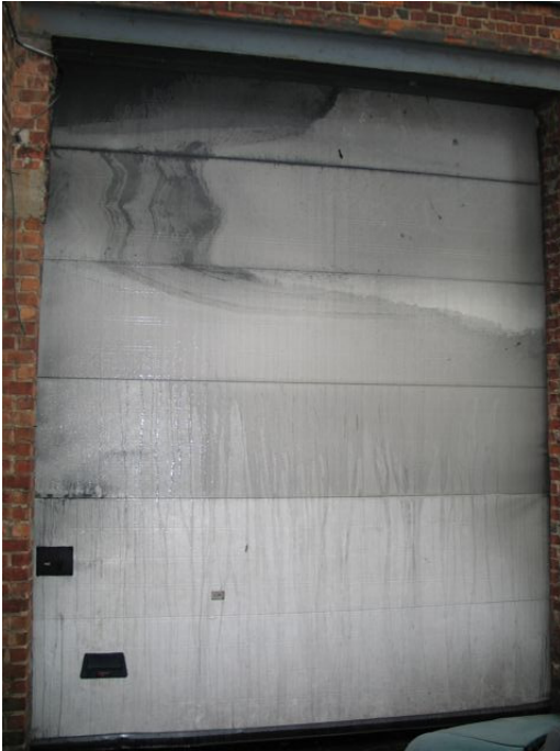
Figure 14 Picture of the garage door taken after the fire. The door has now been forced and was partially in the open position during firefighting. The image that could be seen prior to the first opening has been changed due to water and steam from the extinguishment. Prior to the first opening only the two upper parts were colored due to deposits. The four lower parts were completely clean.
