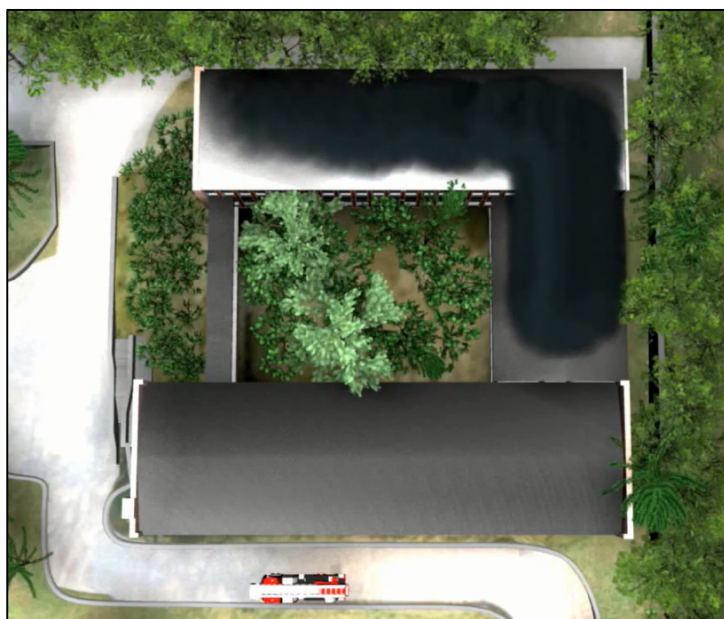
Figure 29 The smoke from building A (up) was going through the void attic space of building C (middle) towards building B (down). (Picture: MSB from [35])
