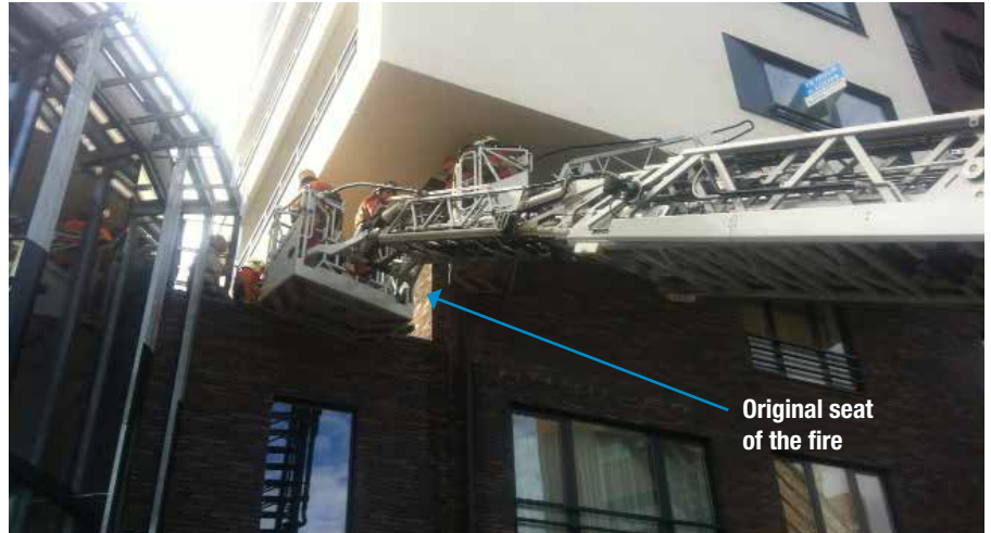
The ladder crew working where the fire started. The section of wall indicated with the bottom blue arrow is about 2 meters wide. The fire could pass the corner and create fire extension across the entire brick wall. Photo by Pieter Maes
